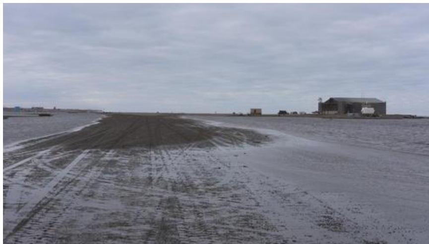
Figure 4. Flooded airport on Barter Island Alaska. Because of the frequency of flooding, the airport had to be moved. Image courtesy of U.S. Geological Survey from https://www.usgs.gov/media/images/flooded-airport-runway-barter-island-alaska .
